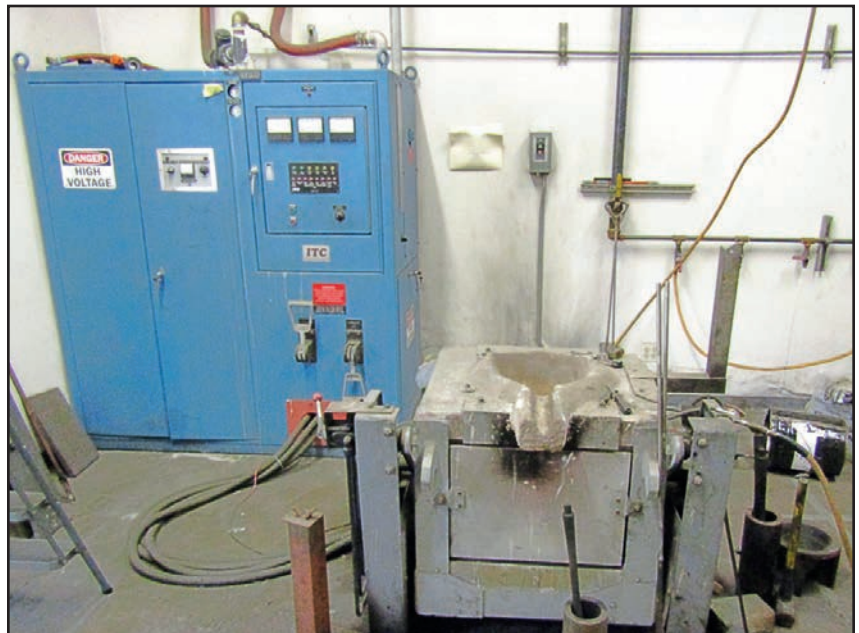
ITC INDUCTION FURNACES W/POWER PACK AND COOLING TOWER
